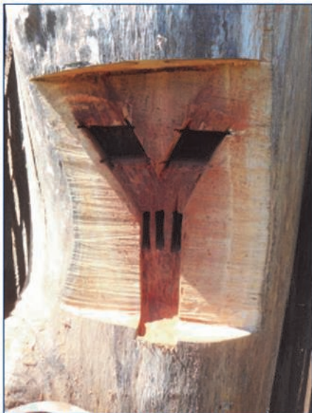
Figure 9 - The bat flats, with the chambers bored out. The idea here is to provide areas of differing temperatures for the bats to move around in as their needs change across the seasons.
