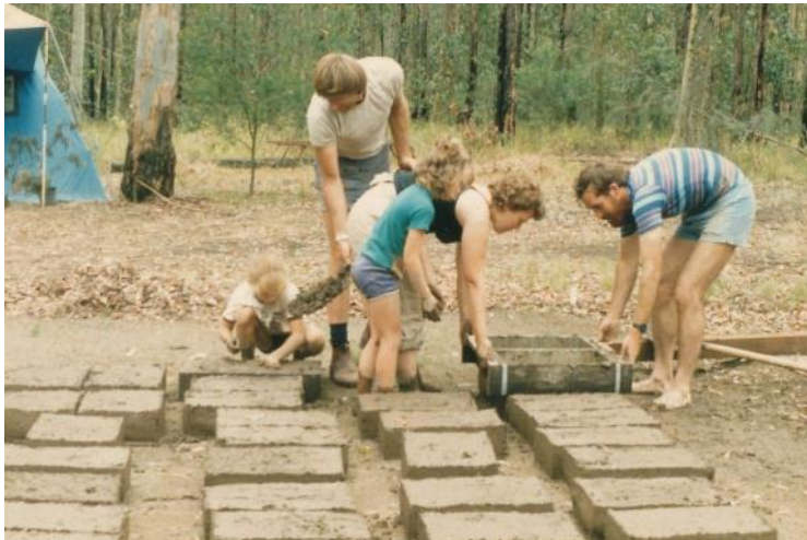
Above: Narawan, Ray, Amy, Wendy and Brian making the mud bricks and Below: the (almost finished) hut.
